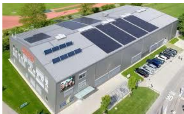
Exterior view of the hall
